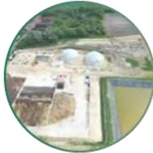
Terrawatt, Marmagne, France
