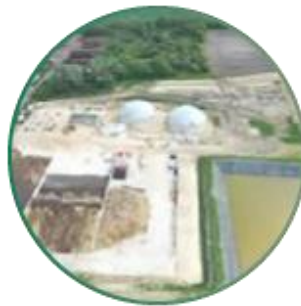
Terrawatt, Marmagne, France
